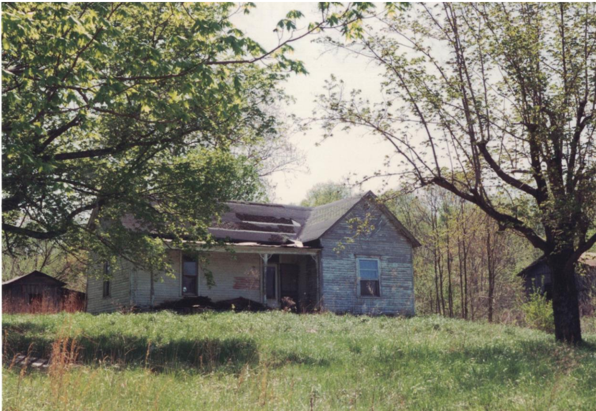
Former home of John H. & Myrtie (Ambrose) Dodson. Photo taken by Jerry Long on 27 April 1993.
