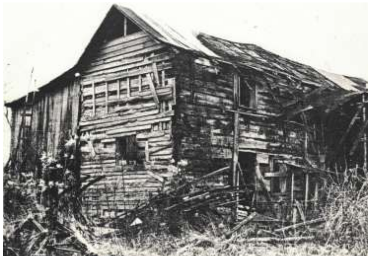
Picture from the Owensboro Star , Owensboro, KY, 4 December 1968, p.1 – “The First Court House in Hancock County is pictured as it looks today. The two-story poplar log house has been flanked by sheds for many years and is still a sturdy structure. It is located near Utility, Kentucky, on the farm of Burtran Ewan. First court held in March 1829, when it was the home of James Dupuy.”
