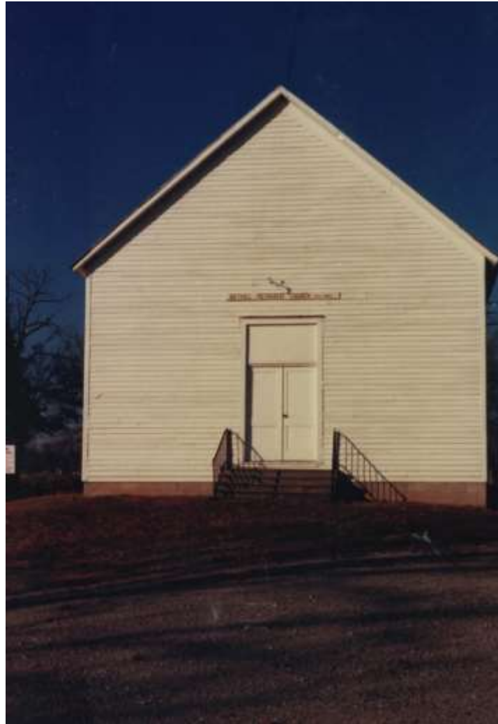
(Old) Bethel Methodist Church Picture taken by Jerry Long On 19 November 1987
