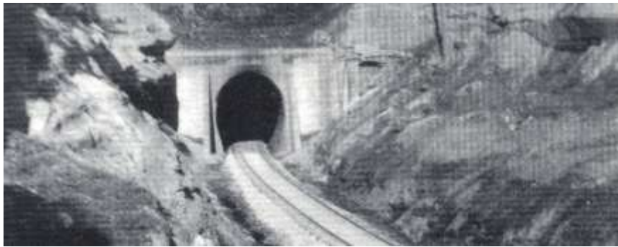
Illinois Central Railroad tunnel at south edge of Rosine
