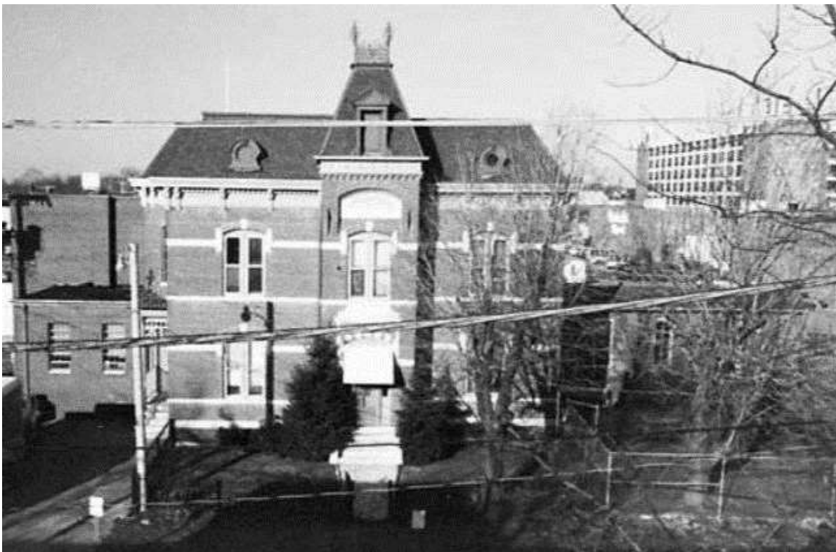
Daviess County Jail, 110 St. Elizabeth Street, Owensboro, KY. The former Executive Inn Rivermont is in background on the right.
