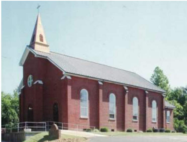
St. Lawrence Catholic Church near Knottsville
