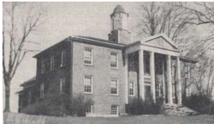
Whitesville Baptist Church. Erected in 1878; annex in 1929. Picture from A History of the Daviess – McLean Baptist Association in Kentucky, 1844-1943 ; Rev. Wendell H. Rone (Owensboro, KY, 1943) p.208.
