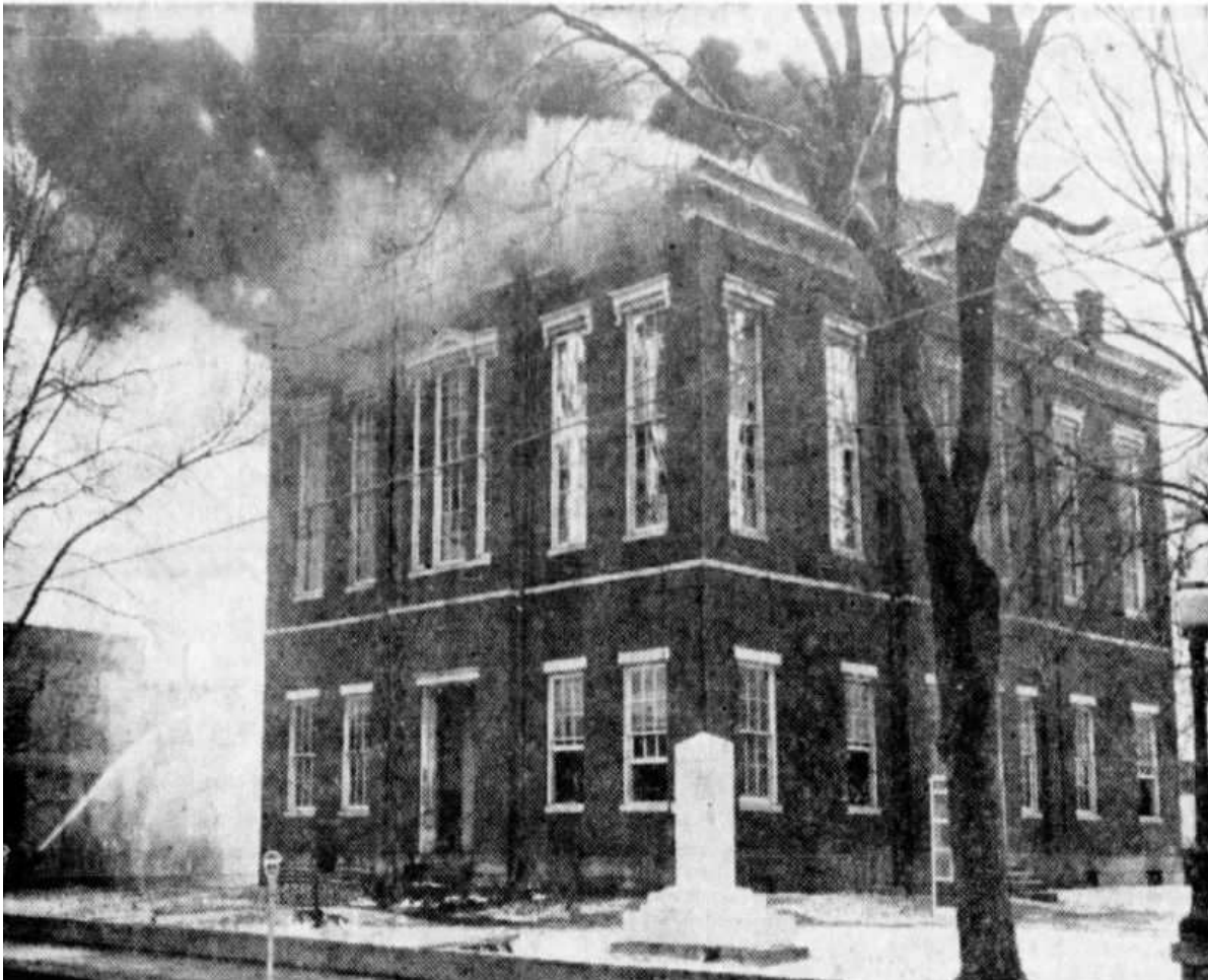
FLAMES shoot from the roof of the 89-year-old Breckinridge County Courthouse as fire destroys the Hardinsburg landmark. Most of the County's records were saved.
