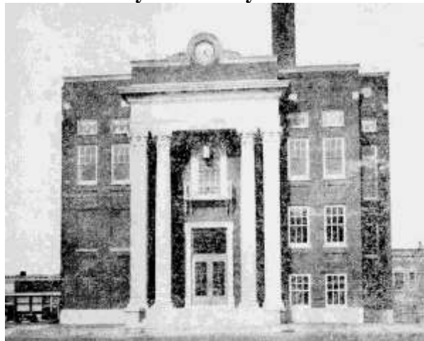
New Grayson County Court House
