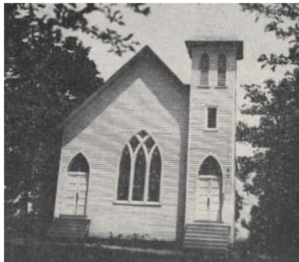
Pleasant Ridge Baptist Church erected in 1906
