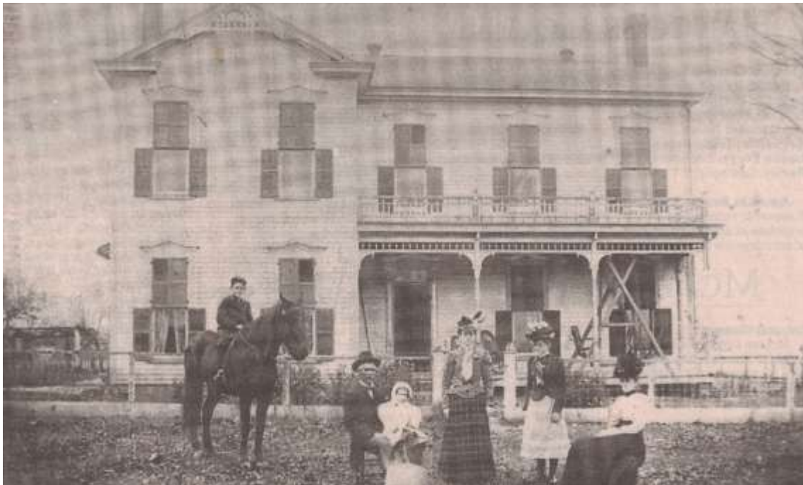
This house stood at Kentucky 762 and Old State Road in Habit. The original building date is unknown, but it was remodeled about 1900. Paul Camp (on horse) lived his entire life in the house, which has now been torn down. The land is currently used as a picnic grove. Photo submitted by Mary I. DeLacey.
