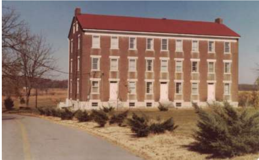
Shaker Wash House constructed by the Shakers in 1854. Part of St. Maur's Priory & St. Mark's Priory 1949-1988. Picture taken by Jerry Long on 11 November 1980.
