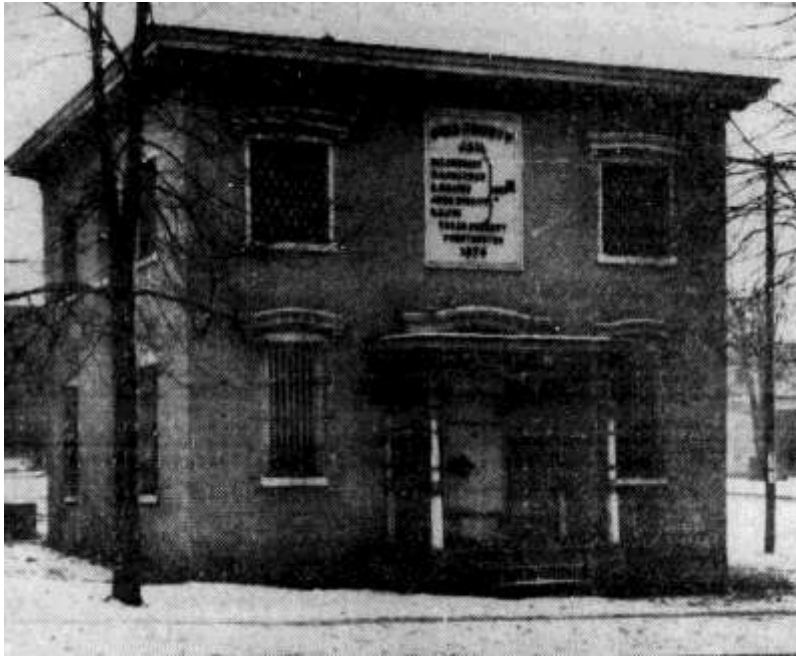
Present Ohio County courthouse at Hartford and county jail
