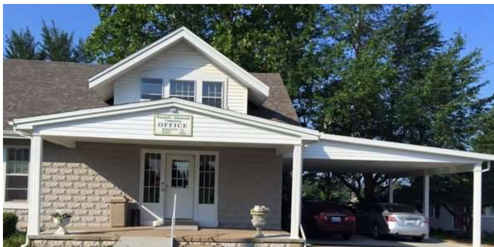
Rosehill – Elmwood Cemetery office, 1300 Old Hartford Road, Owensboro, KY
