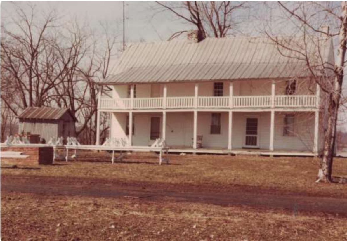
Picture was taken by Jerry Long on 26 February 1980
