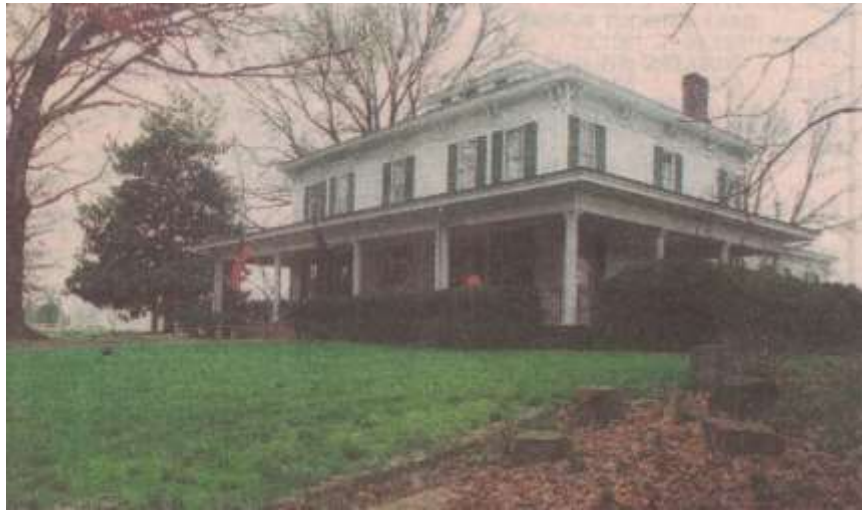
The WeatherBerry home at 2731 W. Second St. will go on the auction block June 29. Bryan Leazenby, Messenger-Inquirer
