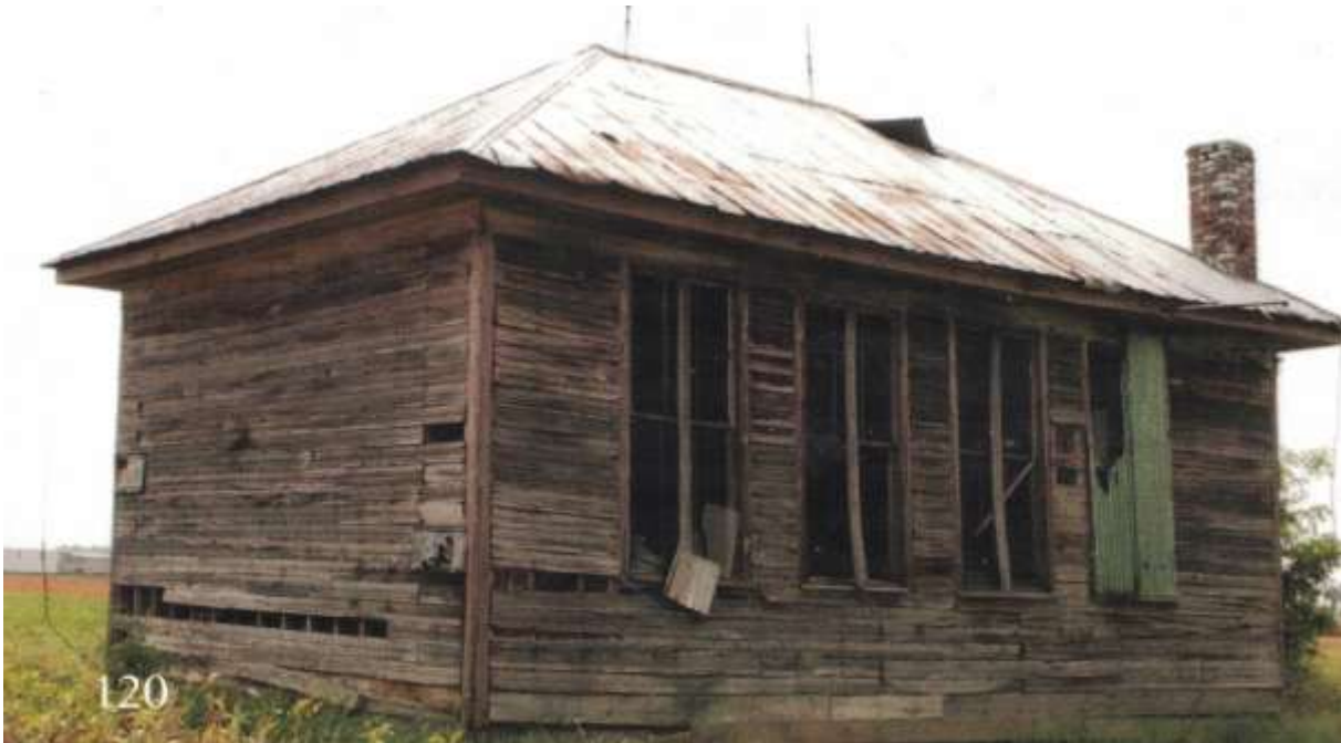
Former "colored" school building in Stanley
