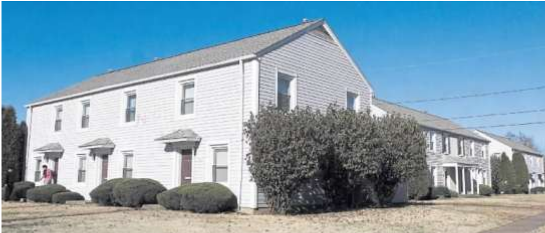
The Nannie Locke Apartments at East Eighth and Jackson streets, owned and operated by the Housing Authority of Owensboro, is in line for exterior upgrades in 2017. Fifty apartments were built in 1954 and dedicated on 16 January 1955. ( Messenger-Inquirer , Owensboro, KY, Saturday, 31 December 2016, p.1A)
